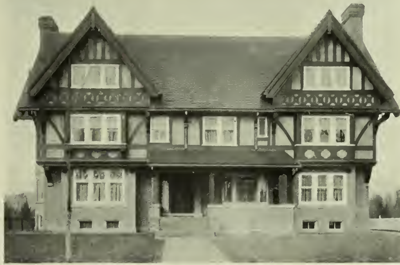
HOUSE AT CLEVELAND, OHIO. Roofed with combination shingle tile made by Ludowici-Celadon Company. Watterson & Schneider, Architects.
